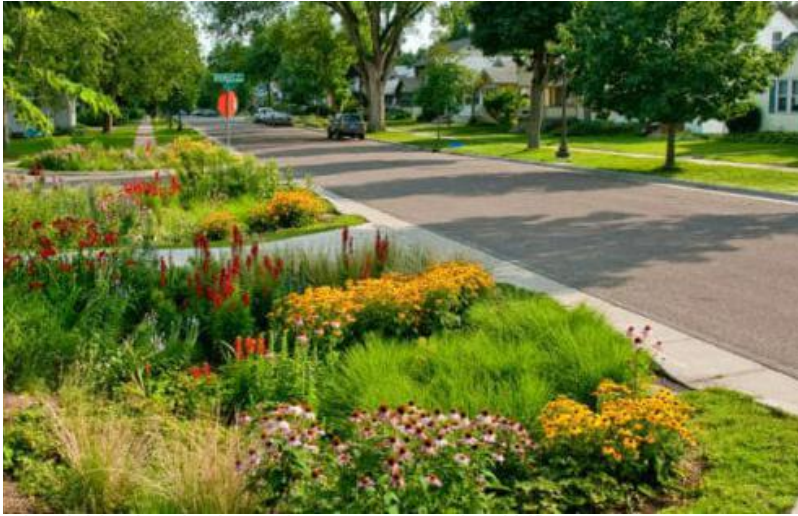
A neighborhood rain garden as an example of LID
