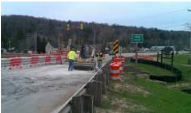
Repair work being completed on the Anna River Bridge
