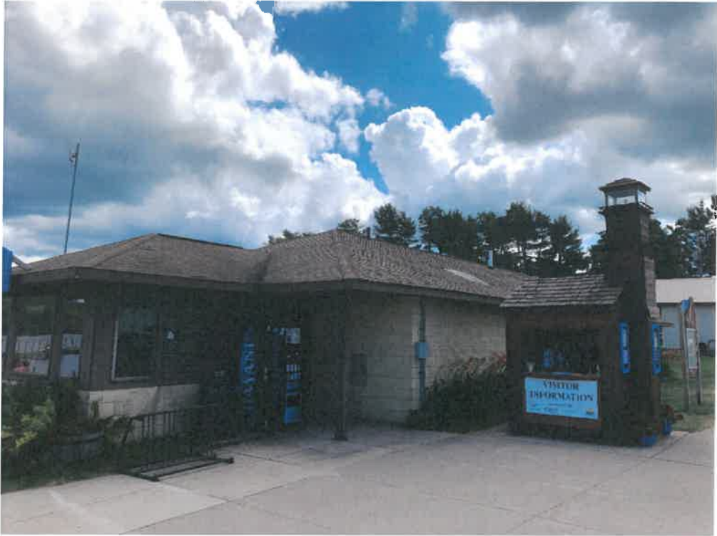
North-West Portion of Building
