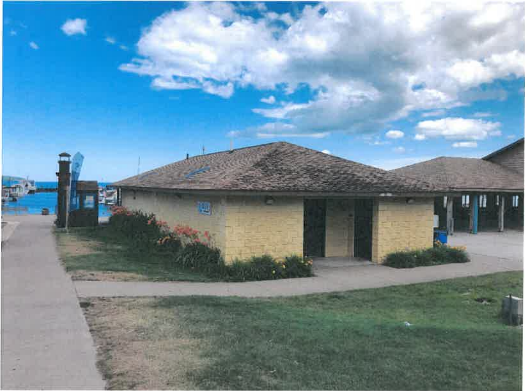
South-West Portion of Building
